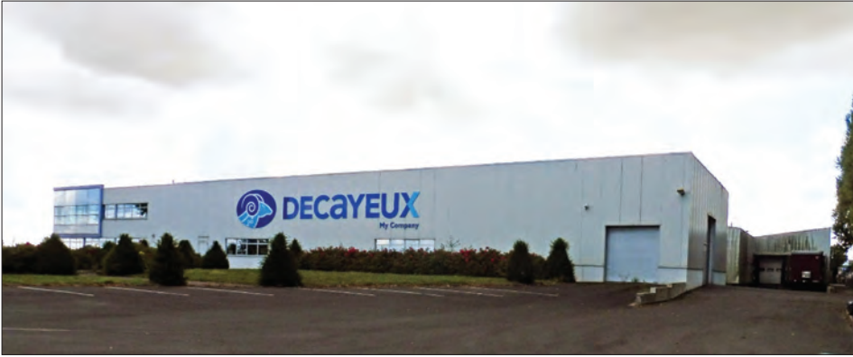
Figure 6. The Decayeux locksmith and small metalwork factory, transferred from the Friville-Escarbotin centre to a functionalist hangar on the Vimeu Industrial Estate (Somme).
